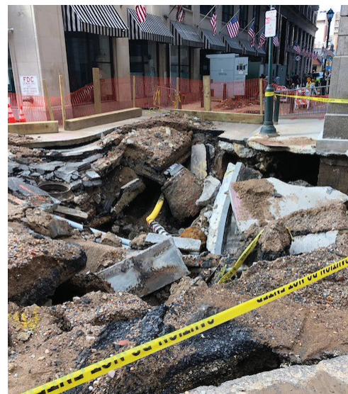
Above: Damage caused by 48-inch water main break
